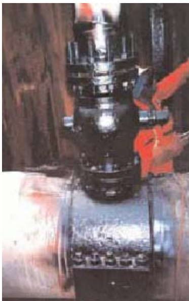
Pictures: Shell Petrol Development Company, Nigeria “Illegal fitting used to siphon crude oil from an SPDC pipeline. One of the two vessels arrested in May 2002 for involvement in crude oil theft. A total of 15,000 barrels of crude oil was recovered by the authorities.” Source: Shell People and the Environment Annual Report 2002, p. 5, by courtesy of Shell Petrol Development Company.
