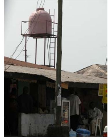
Picture: Max Mader A shop near Eleme. Water tanks are the most common source of water for the sanitary facilities.
